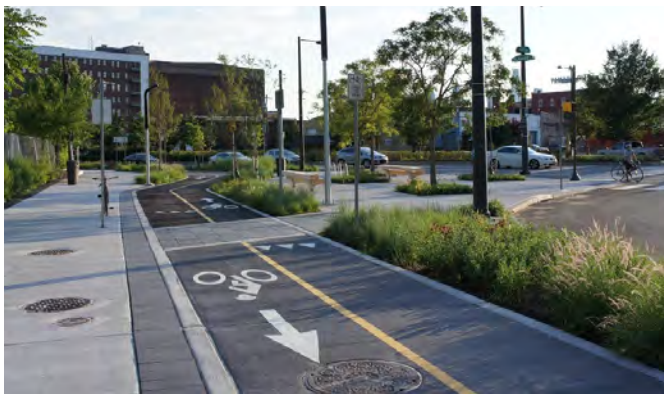
Bike infrastructure like the one shown above provides safe and efficient non-motorized travel, and can serve as green infrastructure to manage stormwater.
