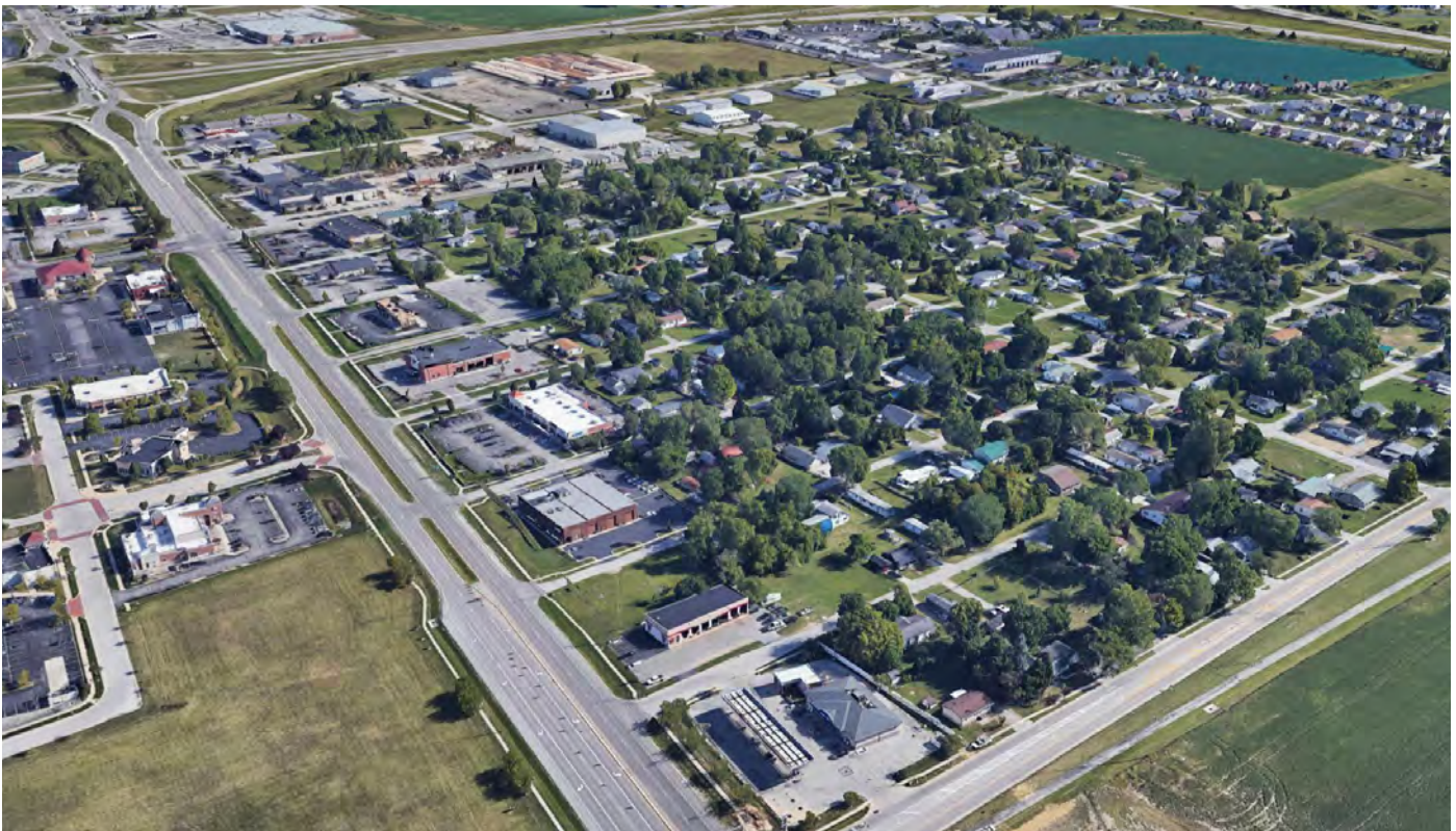
Aerial view of the Heights commercial area fronting Rt. 25.
